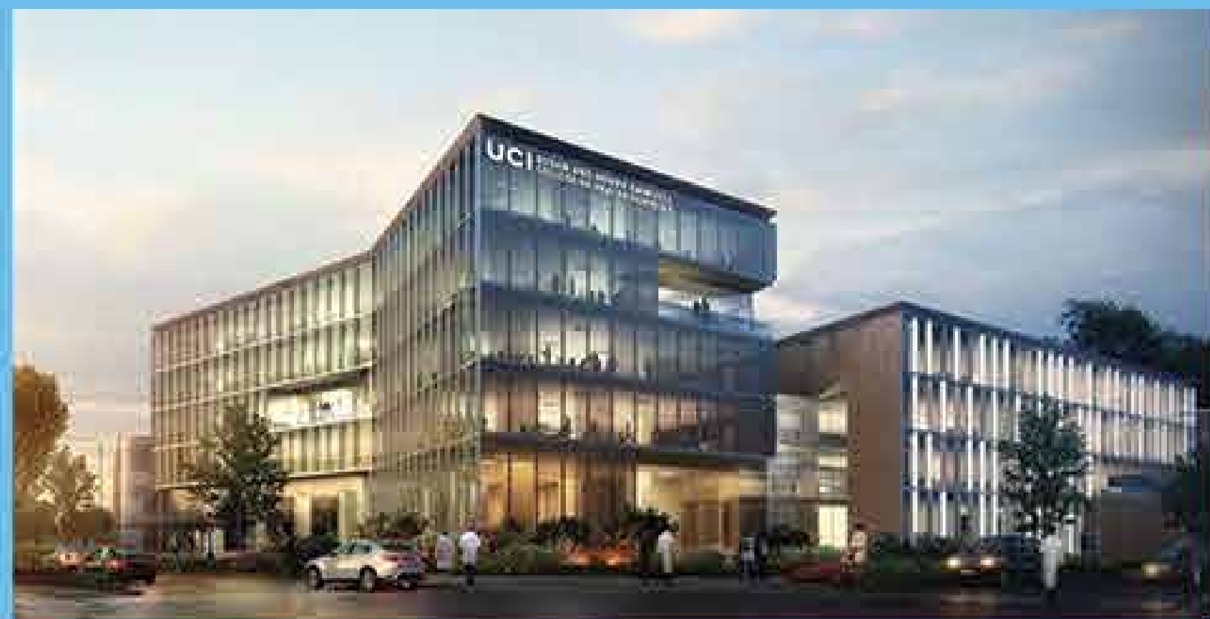
UCI College of Health Sciences Currently Under Construction: Pan Pacific Mechanical & ACCO
